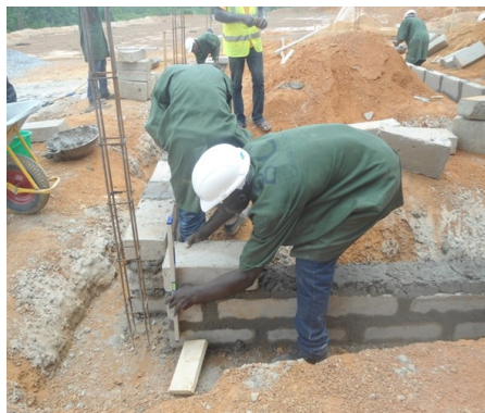
Masonry apprentices during practical work
