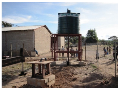
Borehole with header tank, which supplies fresh water to the clinic
